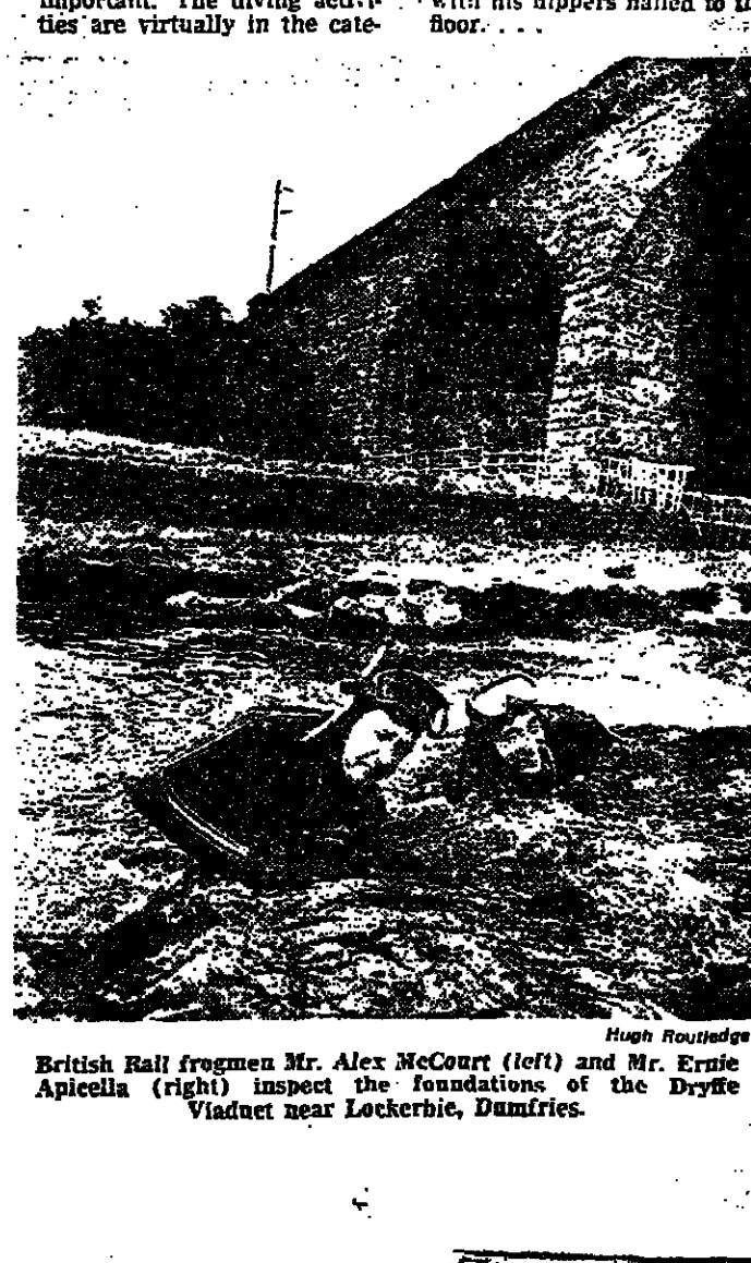
British Rail frogmen Mr. Alex McCourt (left) and Mr. Ernie Apicella (right) inspect the foundations of the Dryde Viaduct near Lockerbie, Dumfries.
